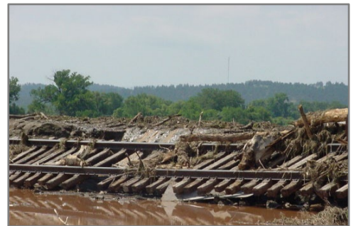
Image 4.7. Aftermath of Aug 2007 flood in Hermosa. DM&E railroad system damage. Image provided by Town of Hermosa.
