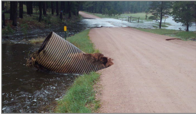
Image 4.1. Flood damage on Lower French Creek Rd. (Image provided by Custer County HWY Department).
